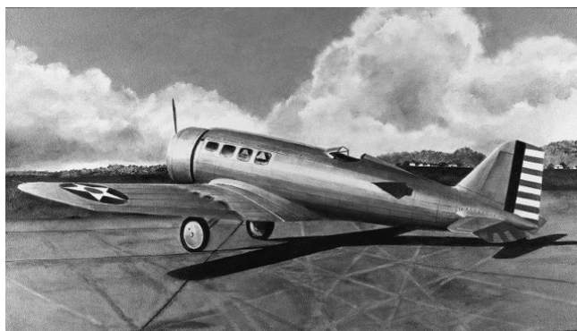
Northrop "Alpha" in USAAC test-aircraft colors. Note the fillet between the fuselage and wing, familiar today and since the 1930s; however, this was the first aeroplane upon which it was featured. Photo circa 1930.
