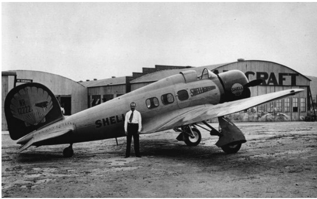
Lockheed "Orion", the last of the single-engine Lockheeds. There is something quite charming about this aeroplane; something both powerful and utilitarian whilst also an artistic aeronautic expression. Note the massive inward-retracting main undercarriage and fully enclosed cockpit (shown open here) Photo circa 1931.
